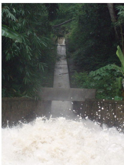
The front view of MHP site of Banjar Arum
